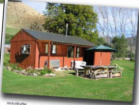
rock crib after
