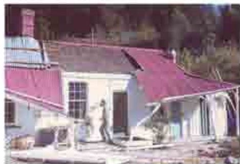
About 1972 a gale force wind lifted the wooden veranda and roof iron exposing the original shingle roof.
