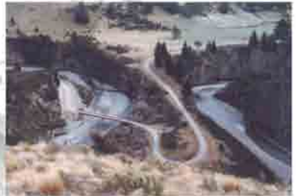
1990's photo looking down on the first bridge as it straddles the previously often uncrossable Mandamus River
