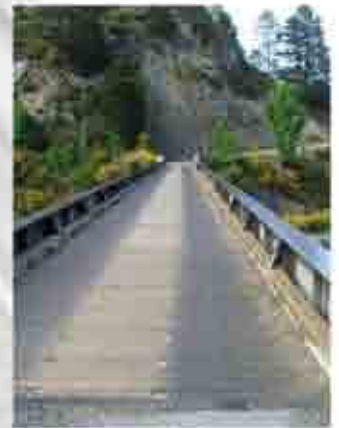
The first bridge 2007.
